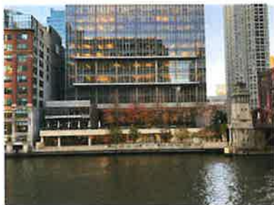
EXISTING - VIEW FROM SOUTH
