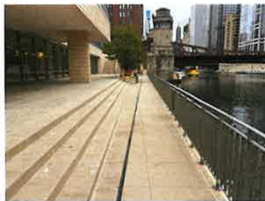
EXISTING - LOWER TERRACE - VIEW FROM WEST
