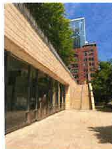
EXISTING - UPPER TERRACE - VIEW FROM WEST
