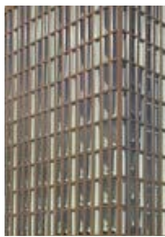
Solid Facade : Facade is articulated with solid metal verticals to break up a window wall system with a solid material at the slab edge and verticals
