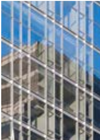
Lighter Facade : Facade is articulated with a higher percentage of glazing with a contrasting color at slab edges and verticals
