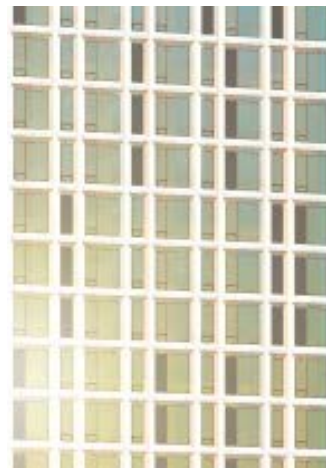
Solid Facade : Facade is articulated with solid metal verticals to break up a window wall system with a solid material at the slab edge and verticals
