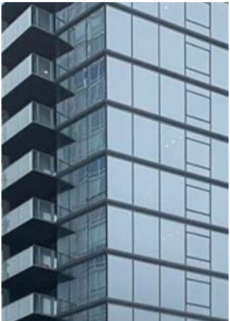
Lighter Facade : Facade is articulated with a higher percentage of glazing with a contrasting color at slab edges and verticals
