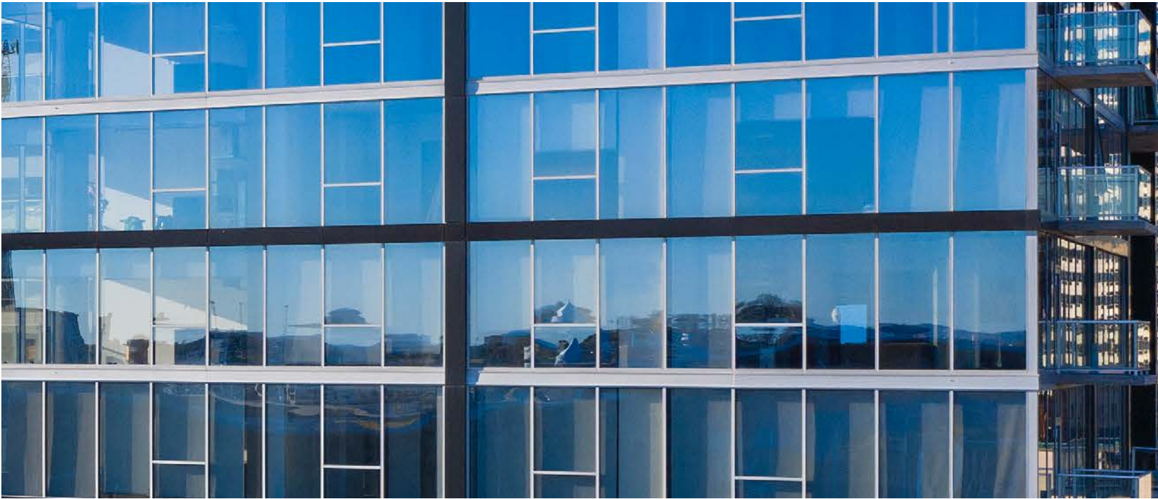
Glass A - Neutral transparent glazing with low reflectivity
