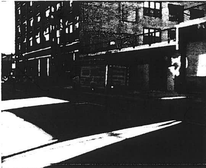
(3) N. MORGAN ST., VIEW SOUTH TO W. WASHINGTON BLVD. & PH II BUILDING.
