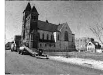
3 SITE PHOTO 3- LOOKING WEST FROM STREET SCALE: N.T.S.
