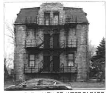
704-06 S. E. 112TH ST. WEST FACADE
