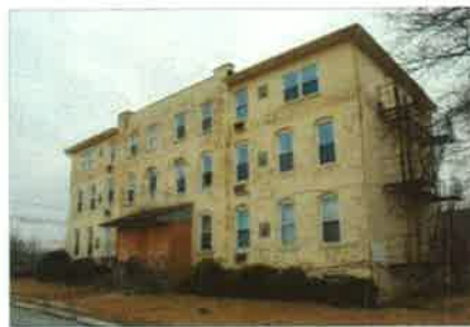
11127-29 S. LANGLEY AVE, FROM SOUTHWEST
