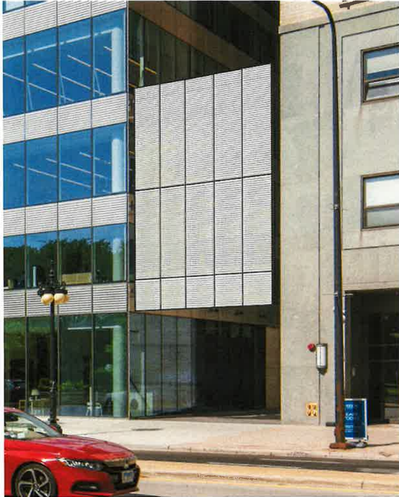
Corrugated Metal Screen to Match Building Facade
