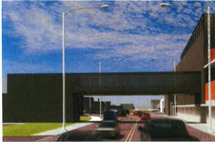
VIEW FROM SOUTHBOUND LANE LOOKING SOUTHEAST
