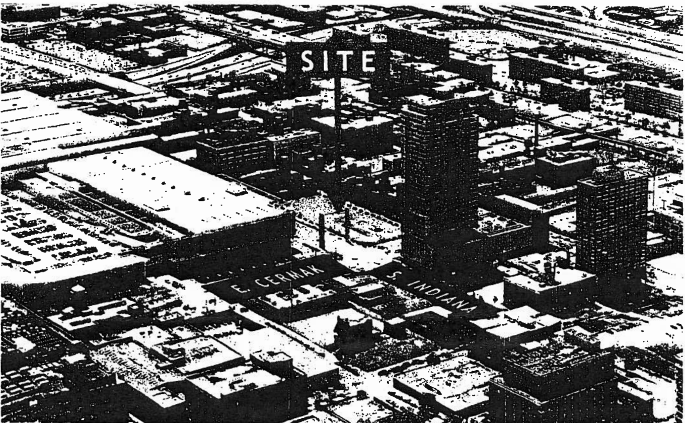
Aerial View Towards Southwest.
